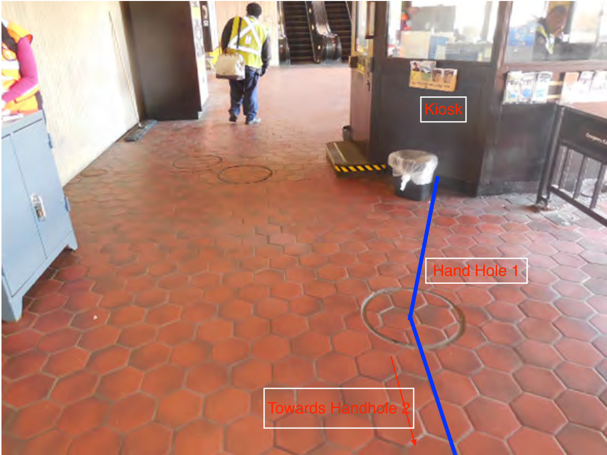
Photo #1 - Hand Hole 1 from Kiosk
